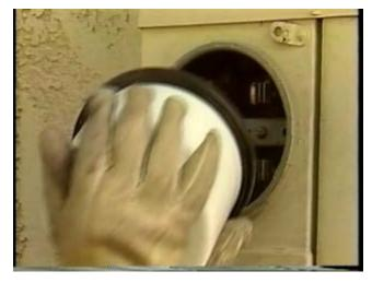
cian then slips a retaining collar over the meter and bolts the collar to the electrical box to secure the meter.
